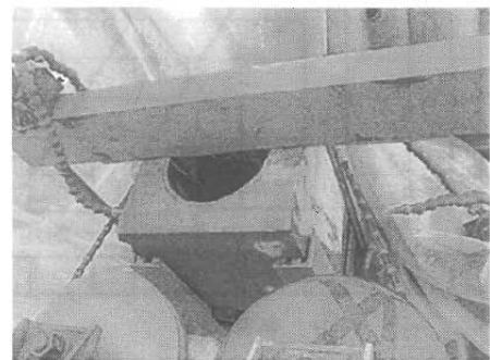
Photo 8 Mortar block (#3) Cutting
